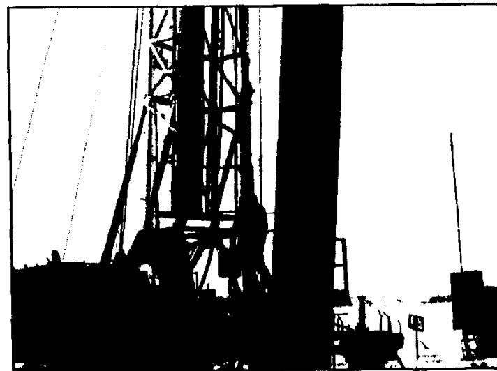
Figure 4 - Service Rig for Installing a TAS® tool - BC
