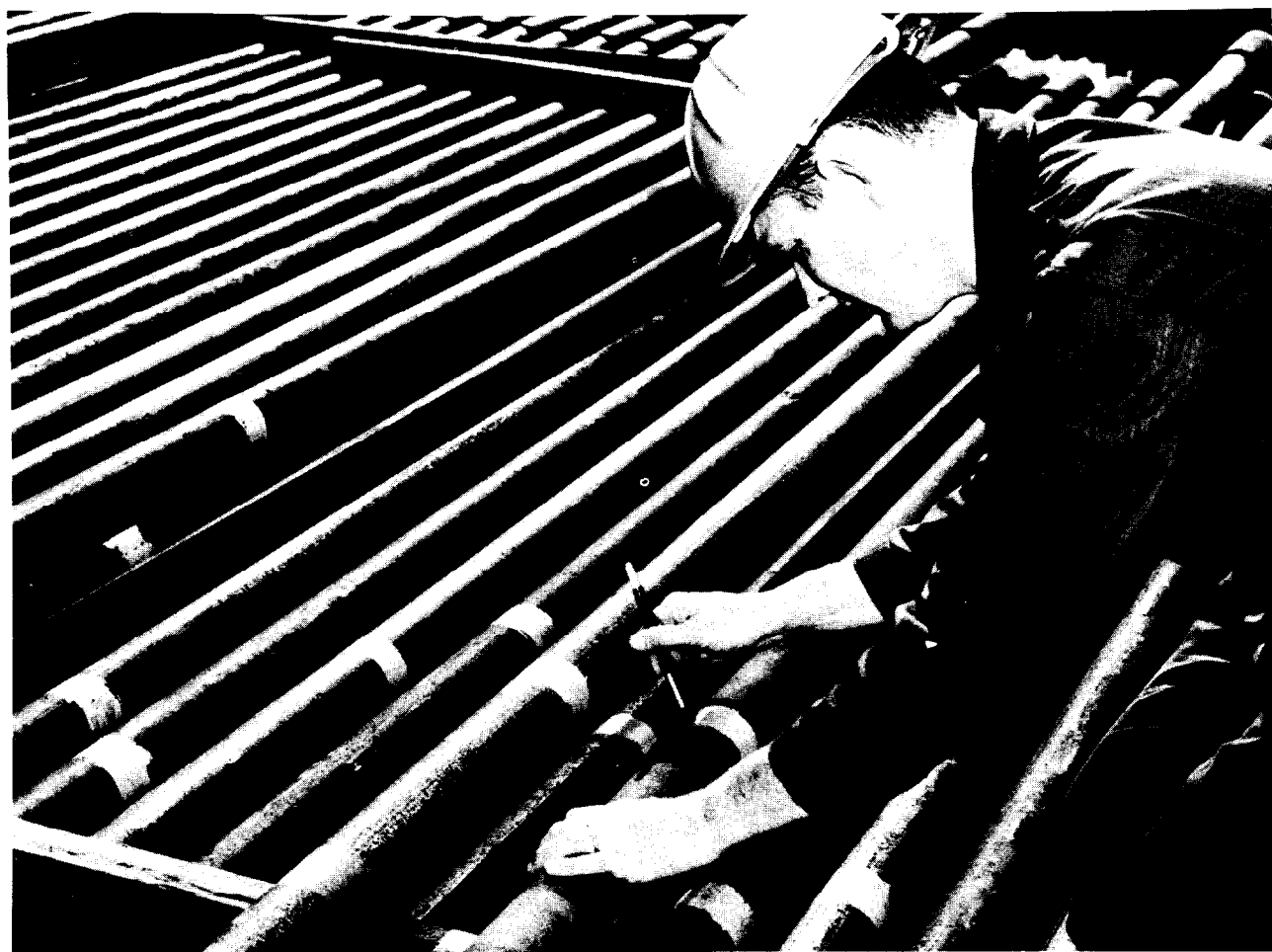
Fig. 8 Color coding used tubing to reflect inspection grade.
