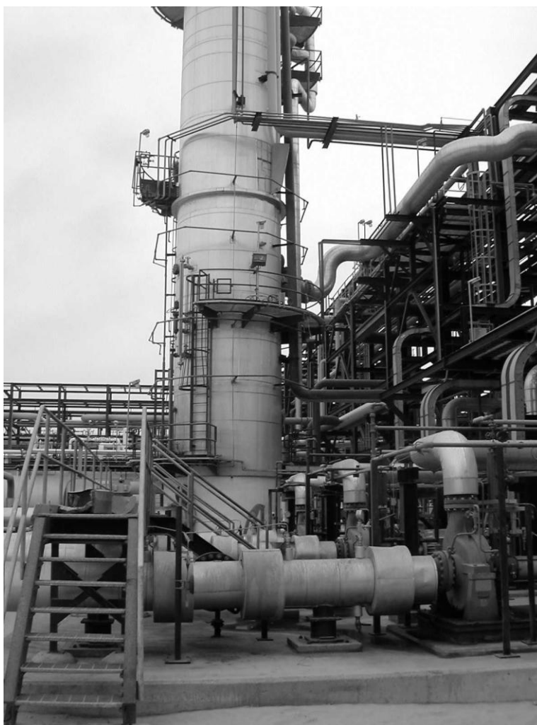
Figure 1 Train 1,2,3 Crude Stabilizer Tower Suction Strainer
