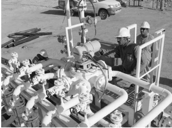
Figure 21 - 3 X 6 X 3 CL 600 Skid Mounted RSV
