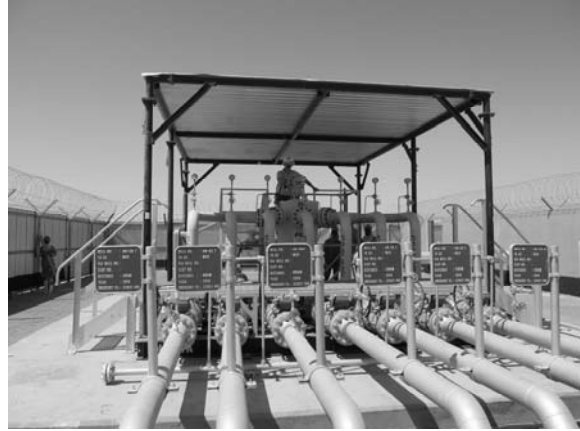
Figure 22 - 6 X 16 X 6 CL 600 Skid Mounted RSV
