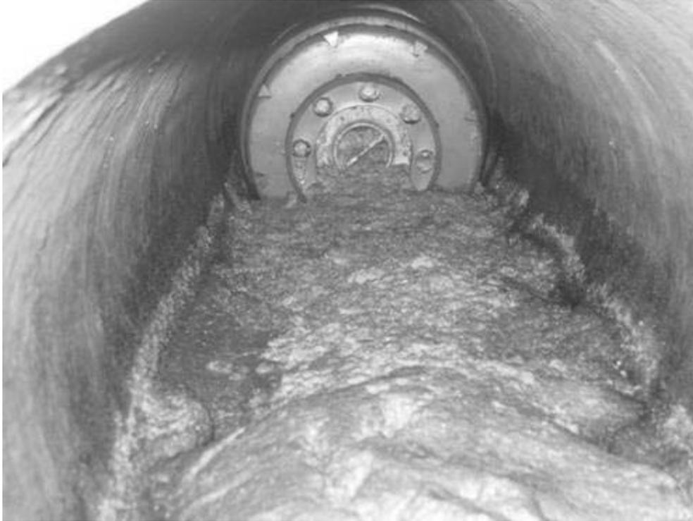
Figure 1 - Rare Photograph of Hydrates Being Removed From a Subsea Pipeline
