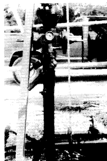
Figure 6a - Example of misalignment between the pumping unit and wellhead assembly
