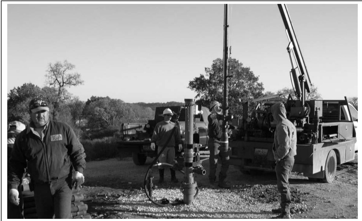
BARNETT SHALE INSTALLATION: Typical well conditions, perforations 8000-8600 feet, vertical. Frac fluid and formation fluid removed by rod pump and tubing plunger.
