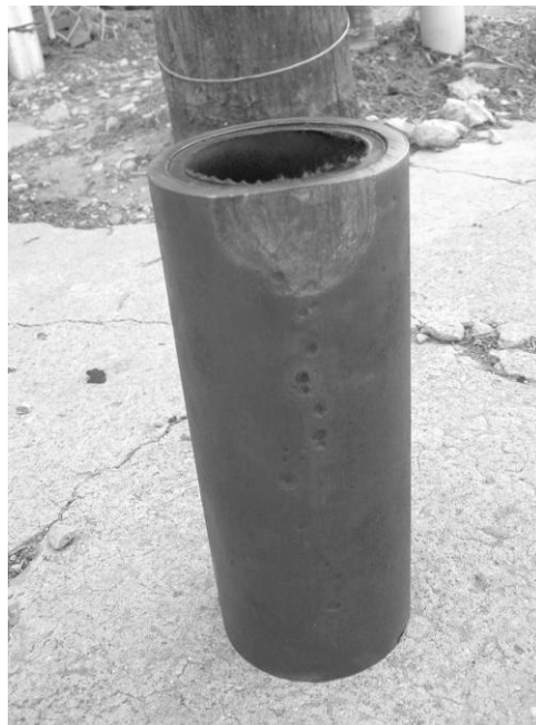
Figure 3 - Bacterial Degradation of Downhole Piping (Yates Petroleum Case Study)
