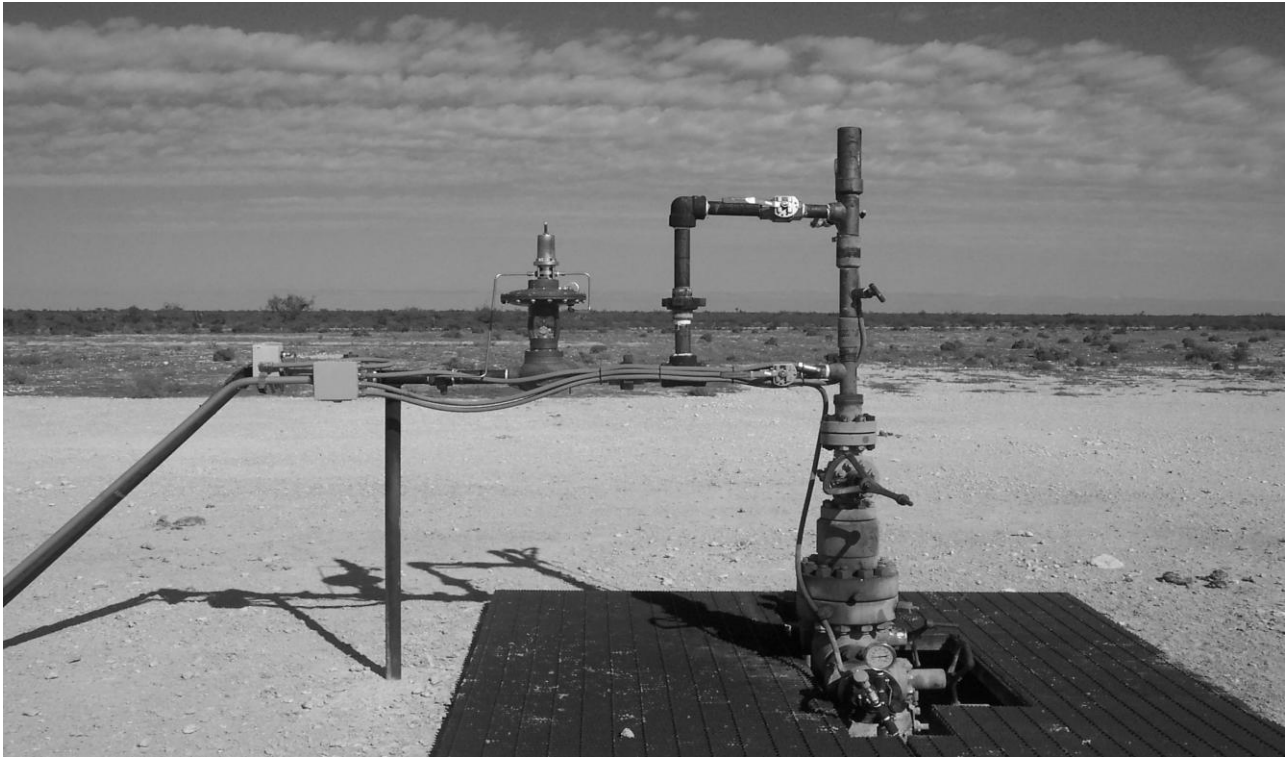
Standard Plunger Lift Installation
