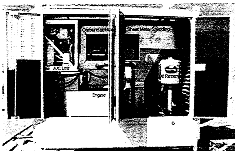
Attachment 6 - View of Interior of Powr/Mastr Unit Showing Engine, A/C Unit, Carburetor, Sheet Metal Ducting and Oil Reservoir
