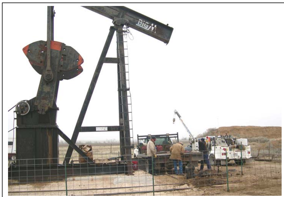
Figure 4 - Ruth Replace 228 Pump Unit with Casing Plunger
