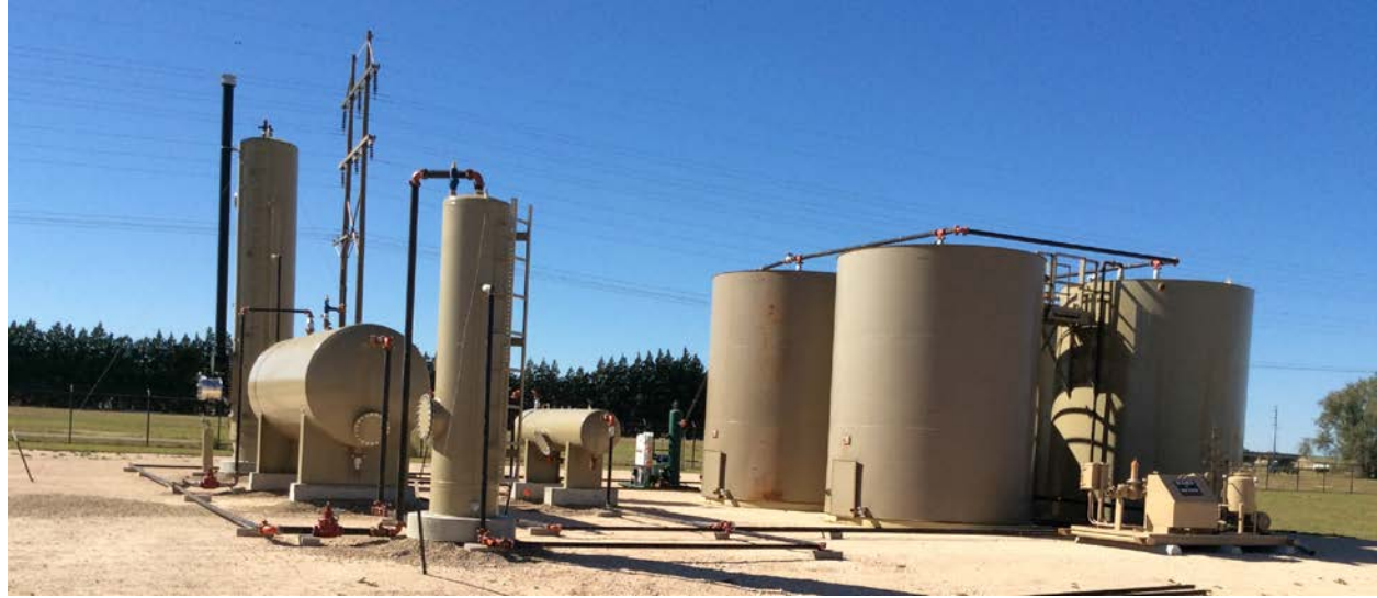
Figure 3 Tank Battery
