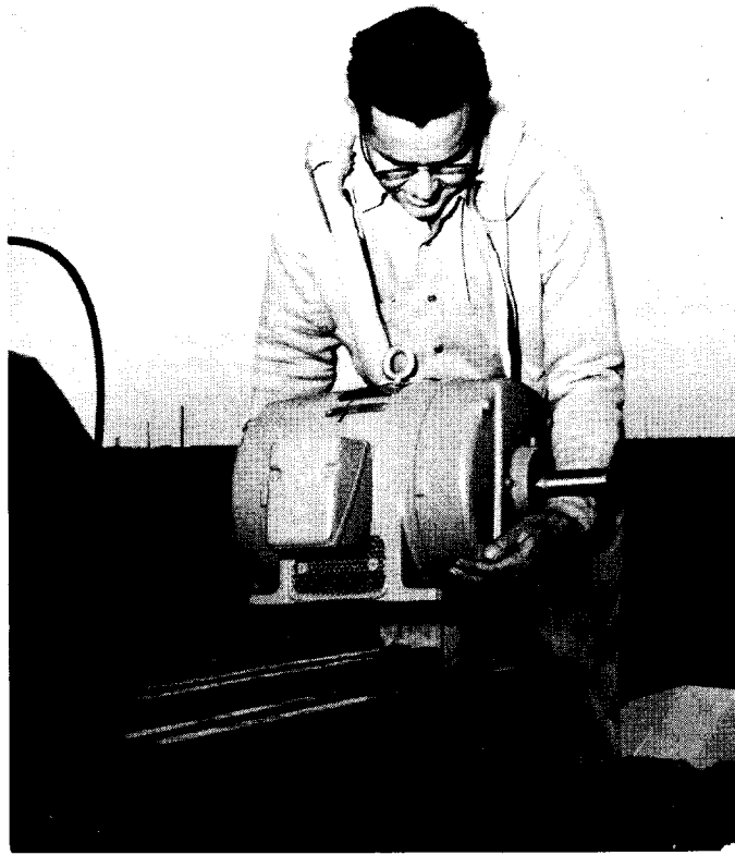
Figure 4. Modern Induction Oil-well-pumping Motor Incorporating Design Improvements and Accessories for Outdoor Use
