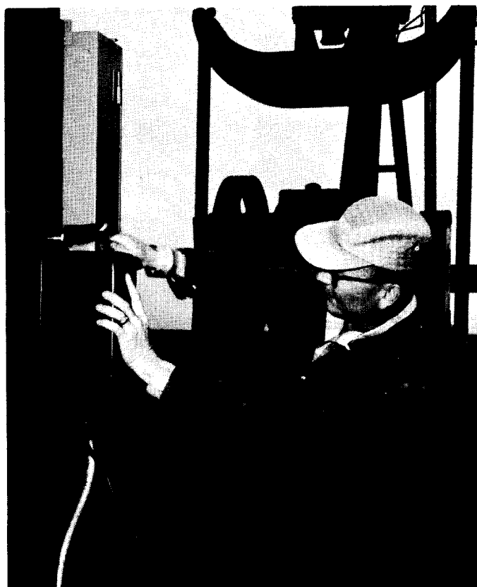
Figure 6. Usual Method of Installing a Capacitor on the Stub Pole with the Controller at the Well Location
