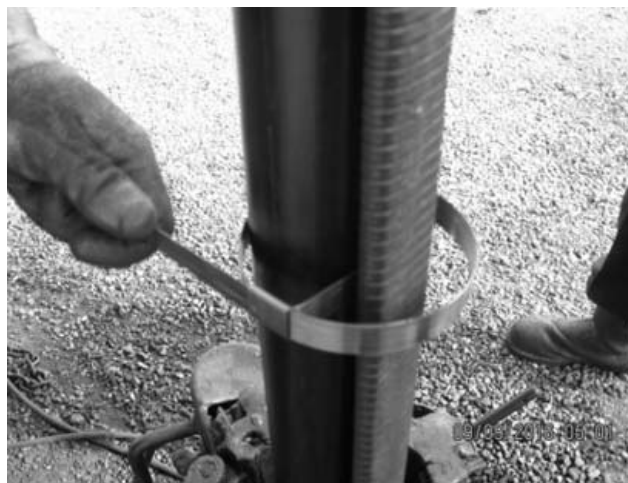
Figure 17: Banding tip. Bend “tang” such it will be under the cable
