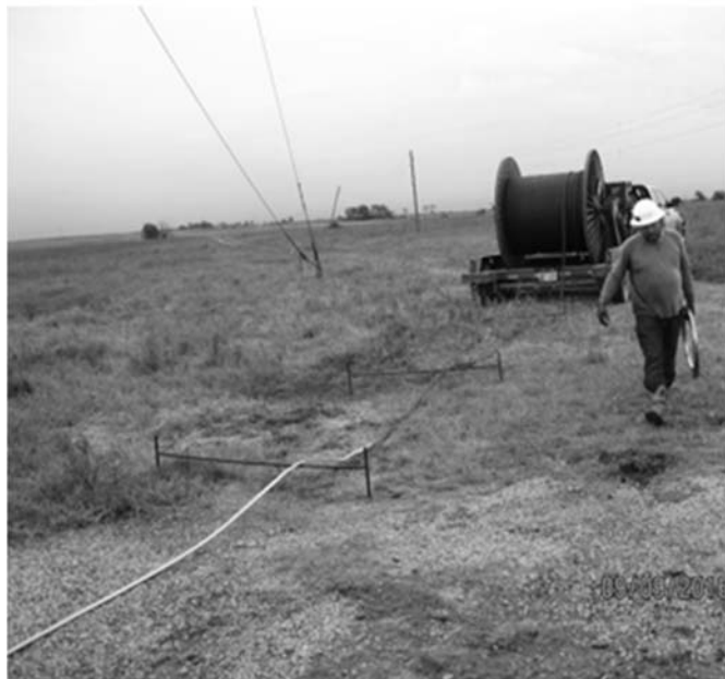
Figure 15: Too few cable supports
