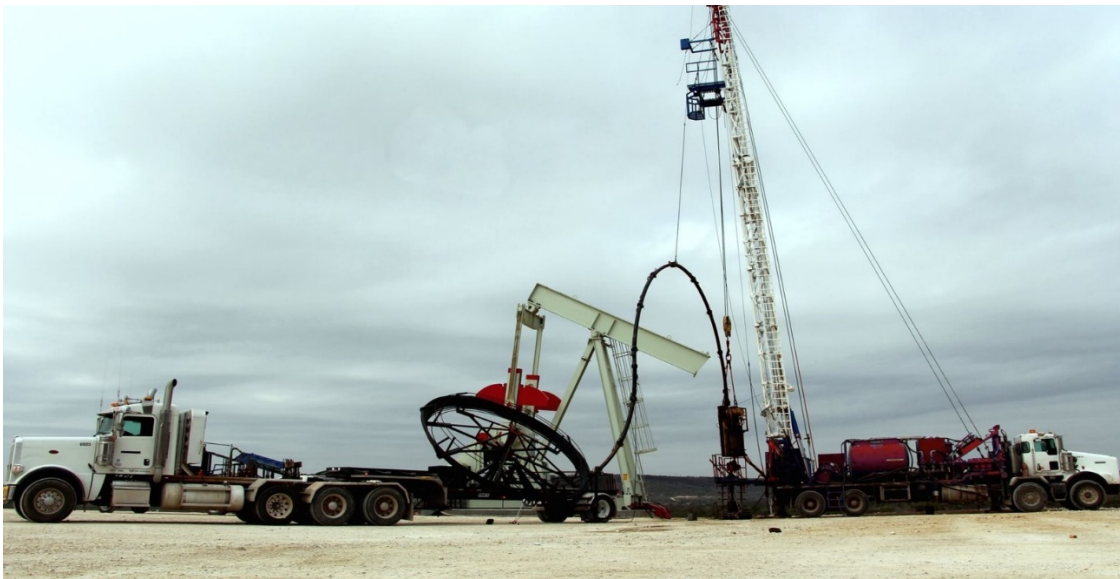
Figure 1: Spooling rig for continuous rod installation
