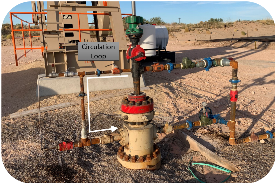
Figure 9 – Circulation Loop, which allows chemicals to be circulated in the well—fluid moves from the tubing to the annulus. These can be helpful in ensuring the chemical gets downhole on flumping wells.
