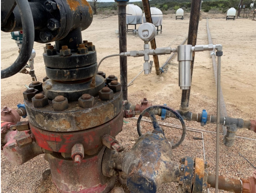
Figure 3 – Capillary String. The Cap String runs from surface all the way to the pump intake downhole and is banded to the outside of the tubing to ensure the chemical can be injected directly into the pump intake.
