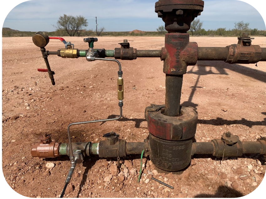
Figure 8 – Clear sight glass on slip-stream. These allow a pumper to visually see if the slip-stream is properly operating and approximate how much fluid is slipping back downhole.
