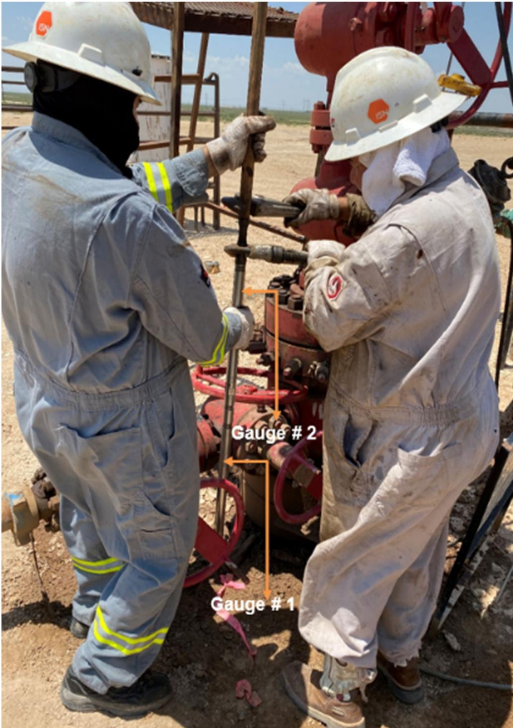
Figure 3: Temperature-pressure gauges with RTD sensors being deployed at the wellsite.
