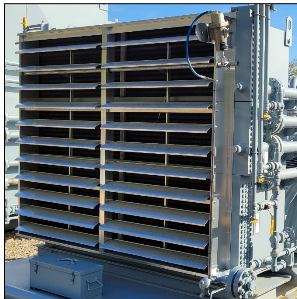
Figure 3 – Electric motor drive gas cooler with automatic louvers
