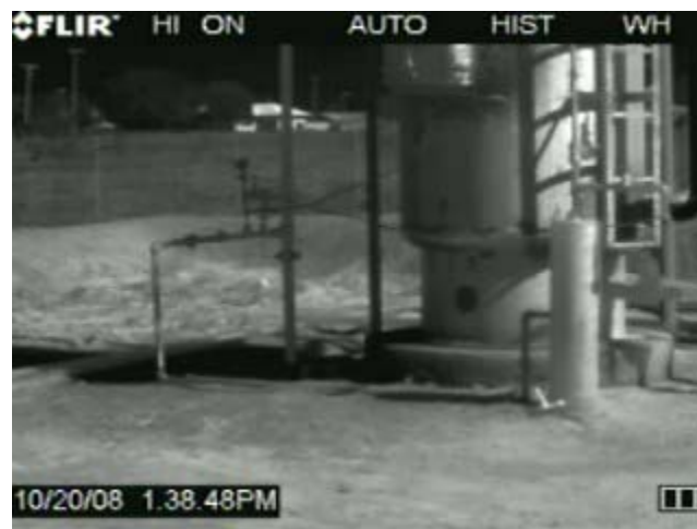
Picture 2 - Same location as above following repair.
