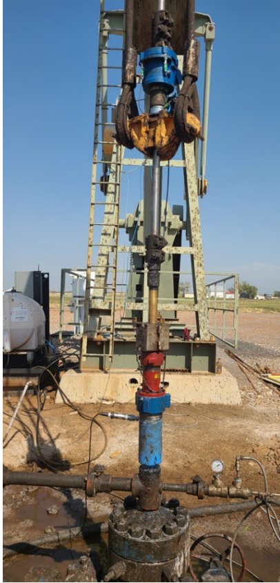
Figure 4 Field test site with stuffing box installed.
