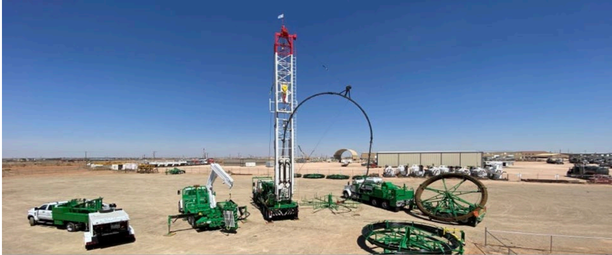
Figure 2—Continuous rod servicing equipment.
