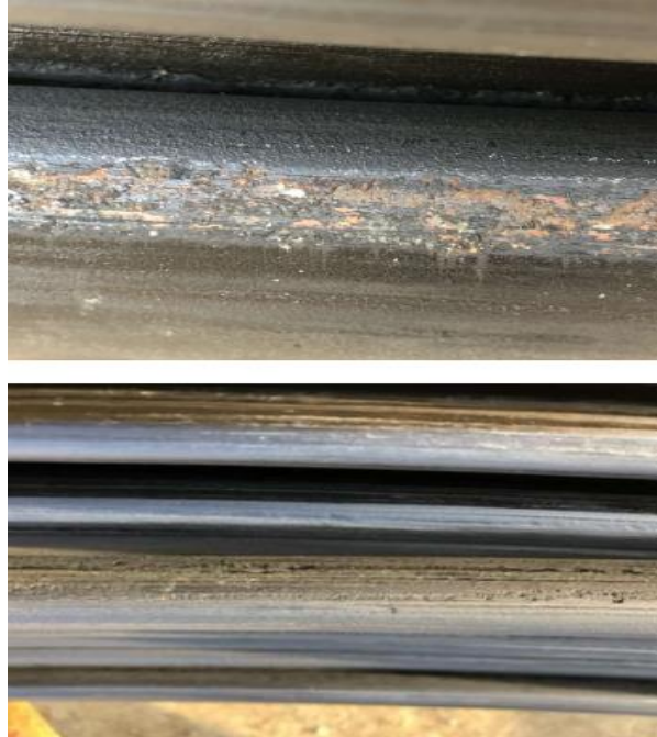
Figure 7: Well No.1 - Moderate Wear
