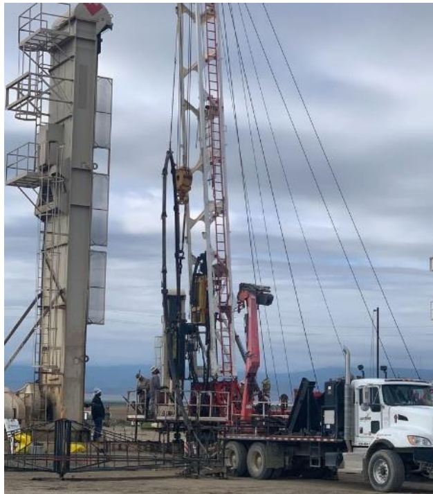
Figure 1: Continuous rod workover operation
