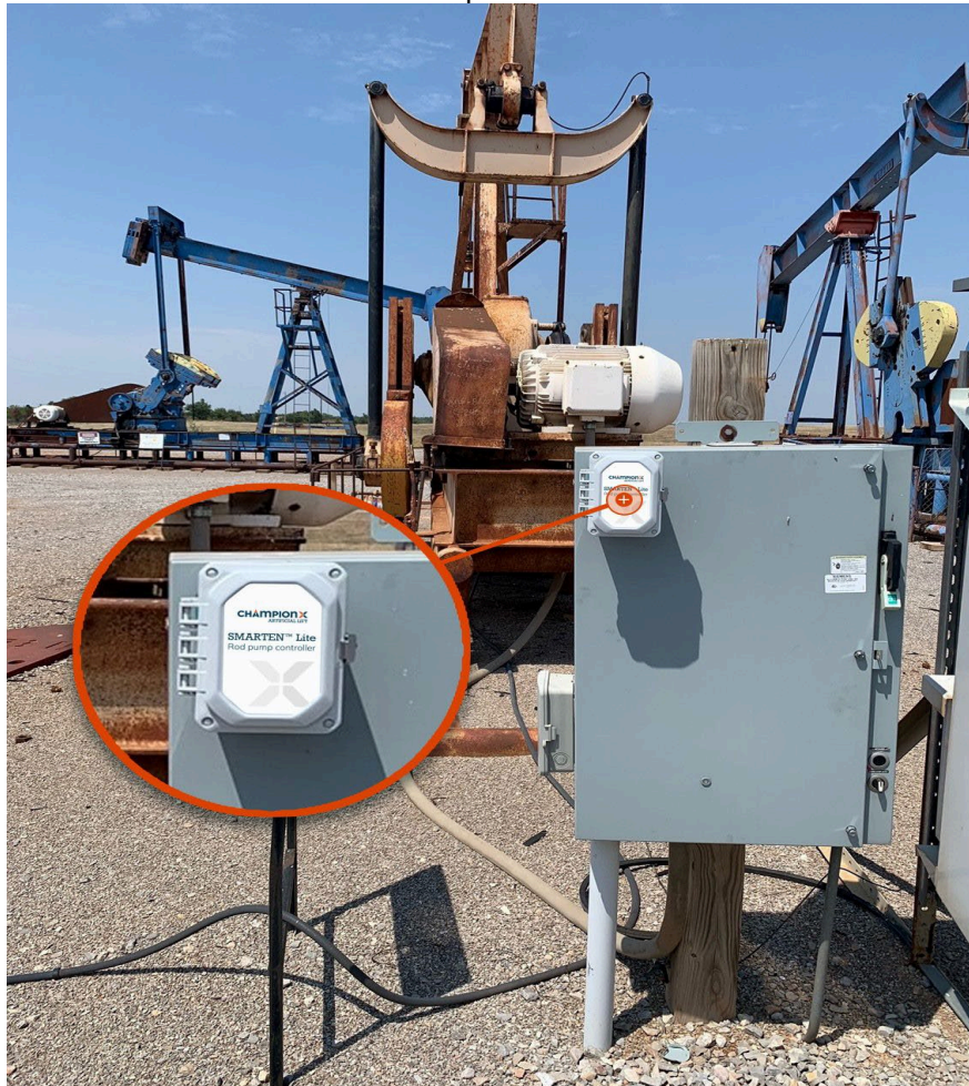
Figure 1 – SMARTEN Lite controller installation
