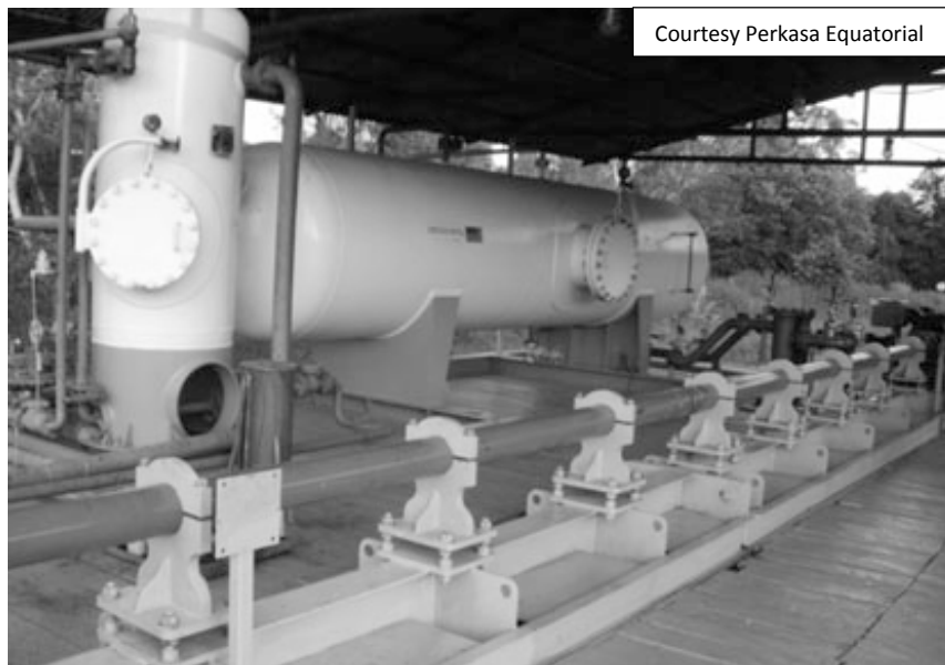
Figure 23.0 Dual Vessel Power Fluid Treatment with Horizontal Pump- 8 years with no failures (PT PERTAMINA 2006)
