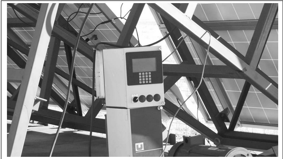
UNICO controller and DC to AC converter
