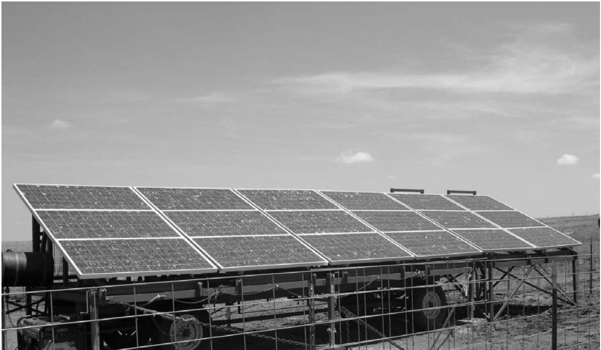
FINAL INSTALLATION WITH 18 SOLAR PANELS WITH 3KW OUTPUT
