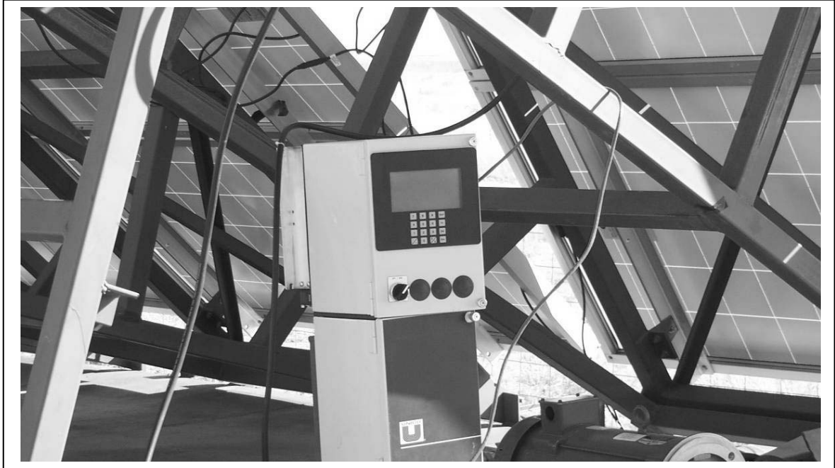
UNICO SOLAR CONTROLLER WITH DC TO AC CONVERTERS
