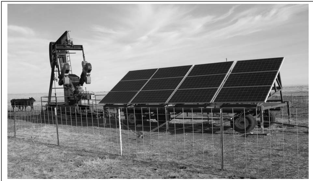
INITIAL 12 SOLAR PANELS WITH 2 KW OUTPUT
