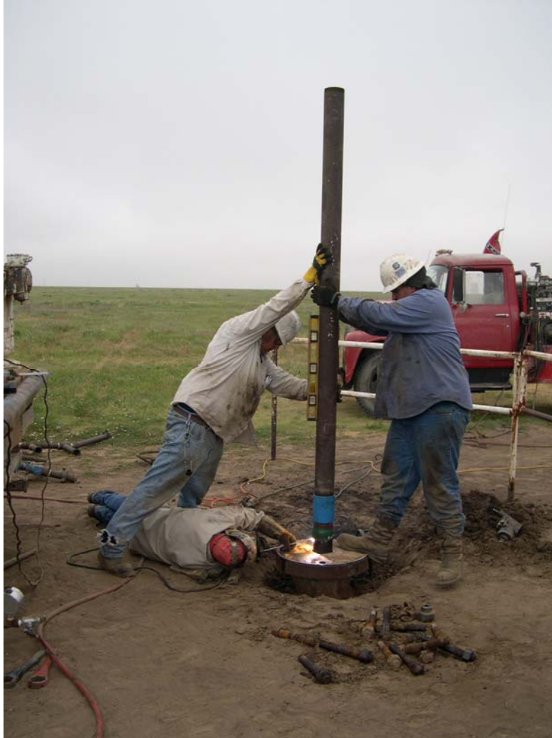
Figure 6 - Bell Nipple with 8 rd Threads Welded Onto Top of Casing Use of vent stack allows gas flow to be safely diverted away from weld site. Alternative flange adapters are available when company policy prohibits use of welding on well site.
