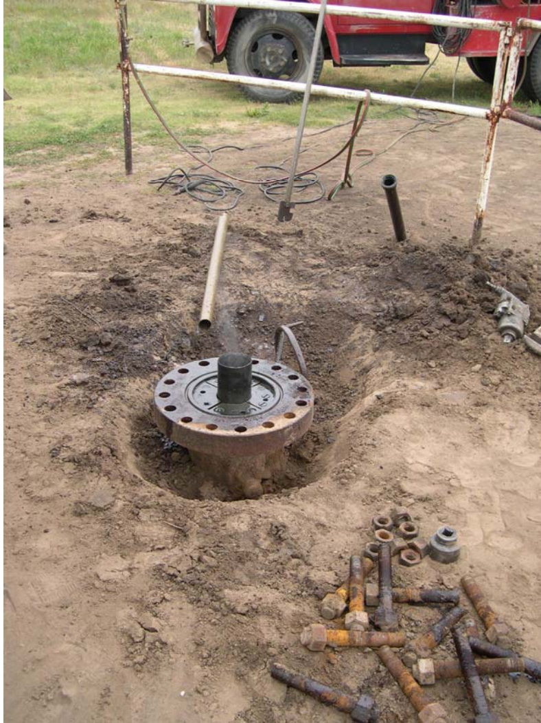
Figure 5 - Top of Casing Prepared to Weld 8 rd Thread Bell Nipple for Full Port Ball Valve Required for Casing Plunger
