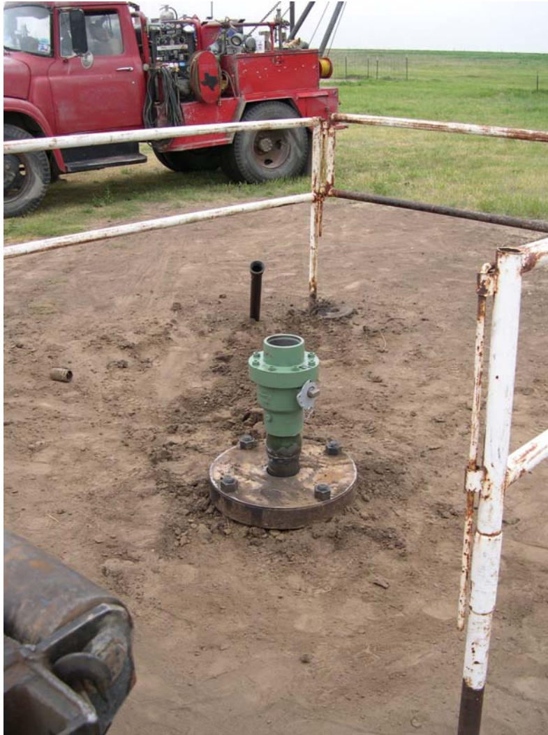
Figure 7 - Casing has been modified for full port ball valve and ready for installation of casing plunger. Should the need arise, the ball valve can be removed and a standard threaded casing/tubing head installed for conventional casing-tubing production applications.
